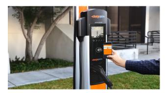
Image depicts a level 2 AC ChargePoint charging station for EVs. (Photo: ChargePoint)
